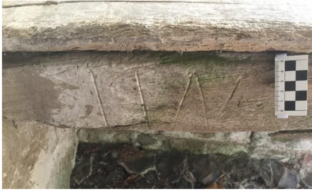
8 Porch interior, east bench, carpenters' assembly marks
